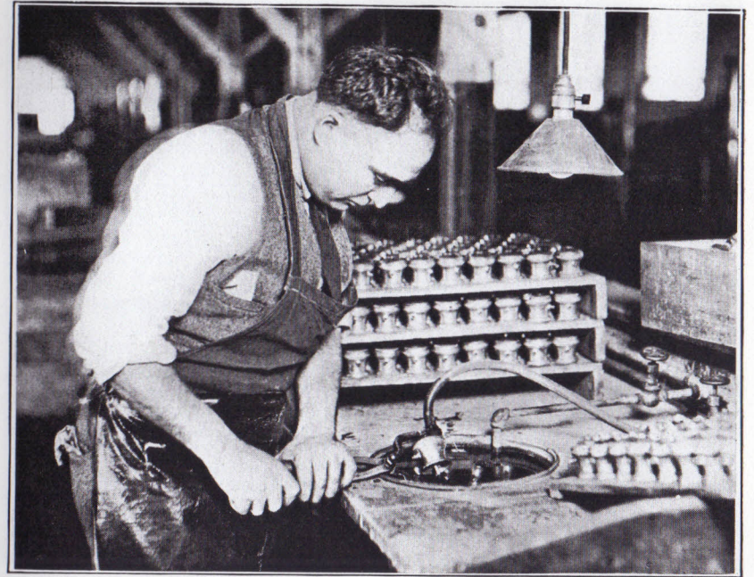
High pressure water testing given to all Auto-Lite carbide lamps.
