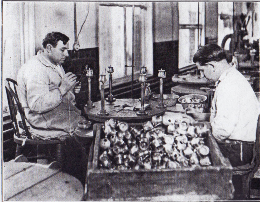
A delicate soldering operation of joining the top cover to the center shell.
