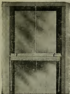
Cut shows position of "Spring Shade," when rolled up. The middle sash makes it practically invisible from the inside.
