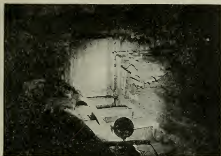
Foundation of Rialto Theatre, Chicago. Illuminated with X-Ray Floodlight
