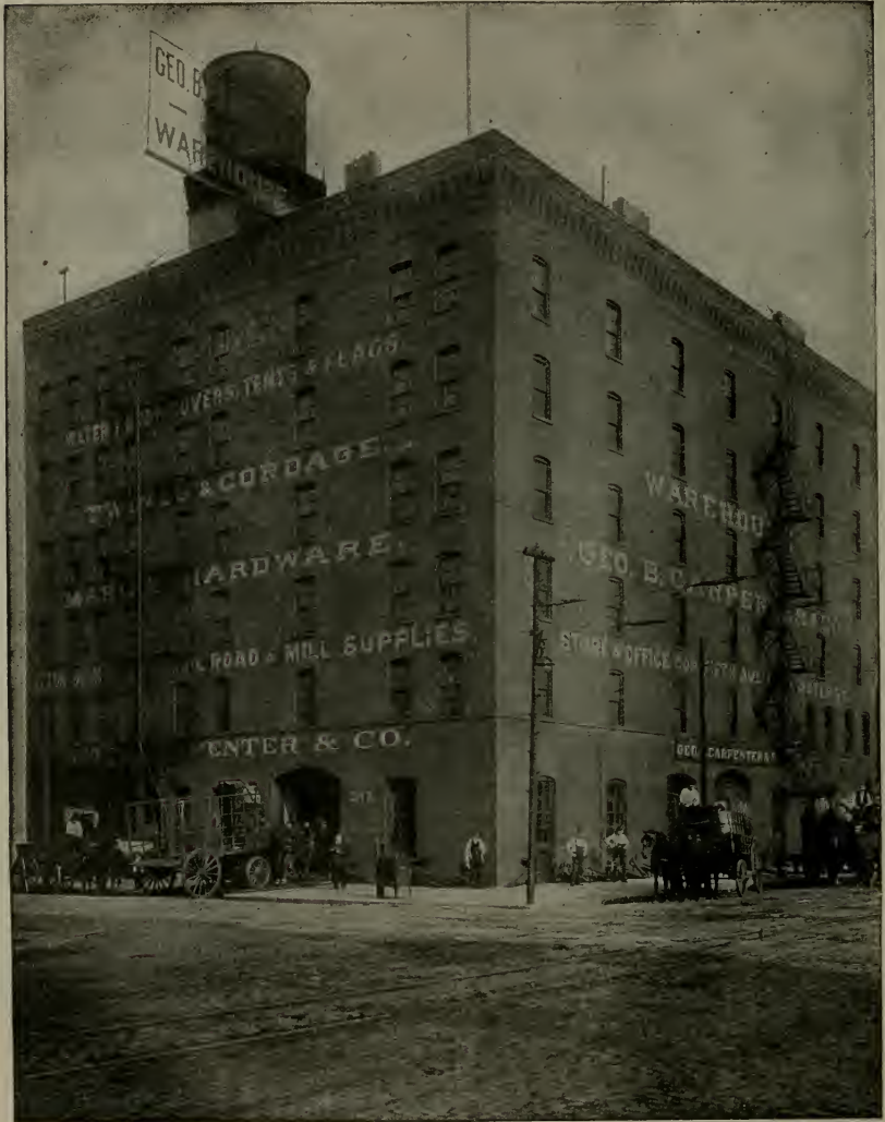
WAREHOUSES A AND B Corner of Grand Avenue and Orleans Street CHICAGO, ILL.
