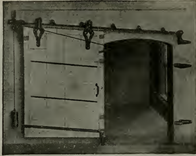
Fig. 500. Inclined Track Automatic Closing Device
